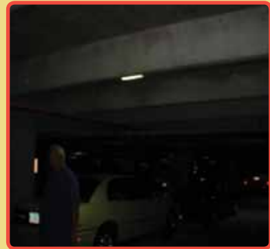
Figure 6.1. Dim lighting in parking area; light fixture is partially obscured by ceiling beams
