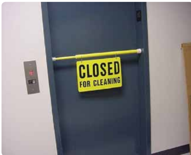
Figure 1.10. Spring-loaded tension bar holds warning sign to block access to room during cleaning.
