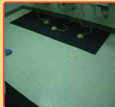
Figure 10.3. Mat is too small, contaminants present on the floor
