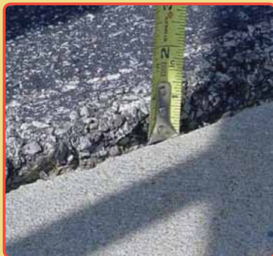
Figure 4.6. Change in elevation (greater than ½") in a walkway outside a hospital building
