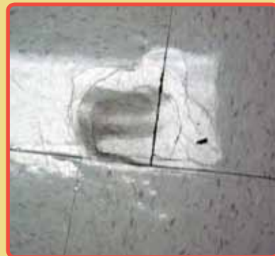
Figure 3.2. Dented vinyl tiles
