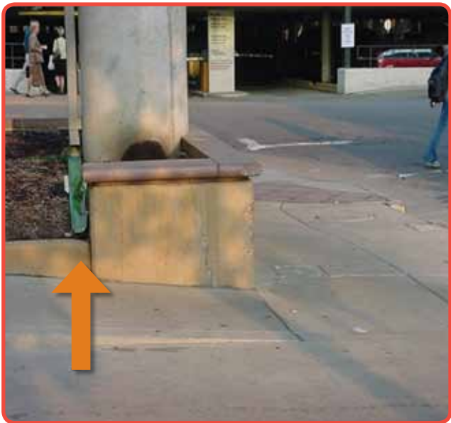
Figure 2.5a. Drainpipe routing water onto a sloped sidewalk (front view)
