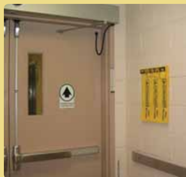
Figure 1.3b. Wall-mounted spill pads
