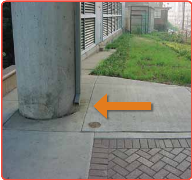
Figure 2.4. Drainpipe routing water onto walkway
